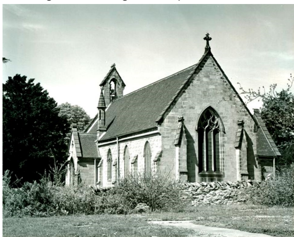
Thorpe Acre Church before the 1986 extensions, image courtesy of Mike Jones
